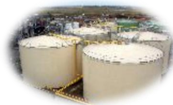
Tanks Farm (Stockage PF + Rétentions)
